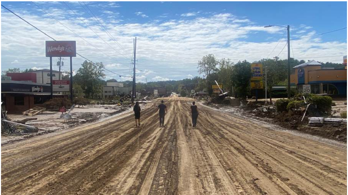
Costs of climate change: aftermath of Hurricane Helene near Biltmore Village in Asheville, North Carolina.
